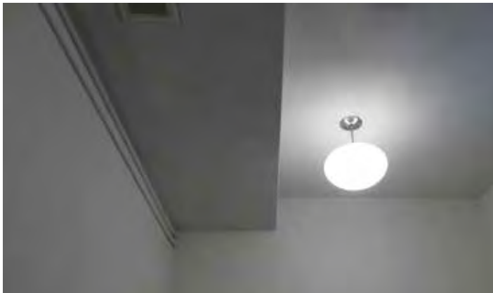
Soffit and exposed conduit in conference rooms adjacent to courtroom
