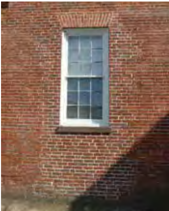
Area of previous masonry patching
