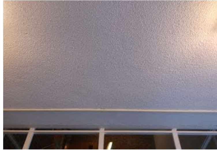
Photograph No. 7 MS Group 2C - White Textured Ceiling Plaster - 1960s Section
