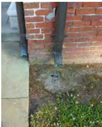
Rain leaders discharge at base of north wall of historic courthouse
