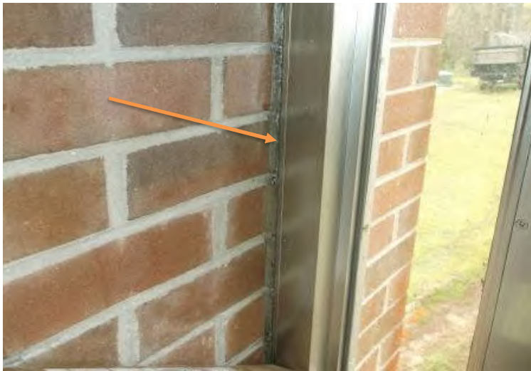
Photograph No. 6 MS Group X - Gray Interior Door/Window Caulk - 1960s Section
