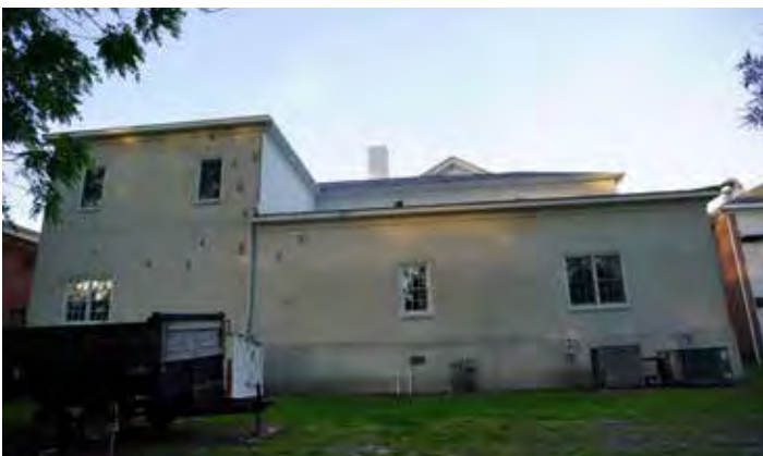
Painted EIFS (dark spots are patches) at 1990s addition
