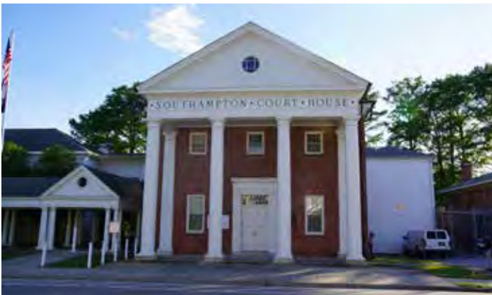
Brick masonry at historic courthouse
