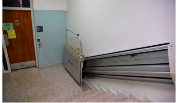
Inclined platform lift provides accessible access to Circuit Court Clerk's offices and Records Room
