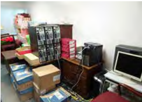
E.27 – Computer servers, Upstairs Conference Room 2
