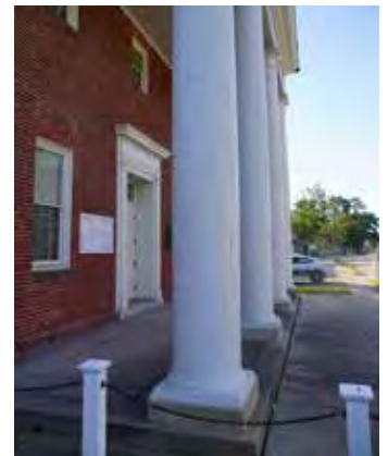
View of portico from SE corner
