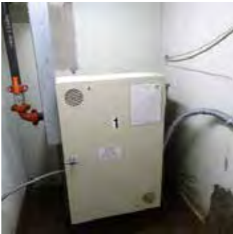
E.23 – Montgomery KONE Elevator #1, 40HP motor
