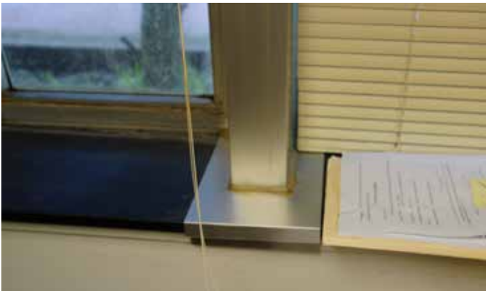
Aluminum cover bridges gap between sill materials where partition previously removed
