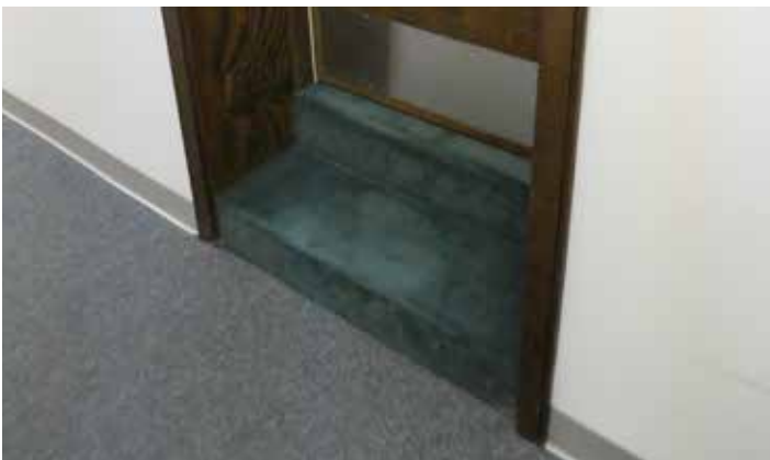
Steps from secure corridor to non-accessible judge's bench in second-floor courtroom
