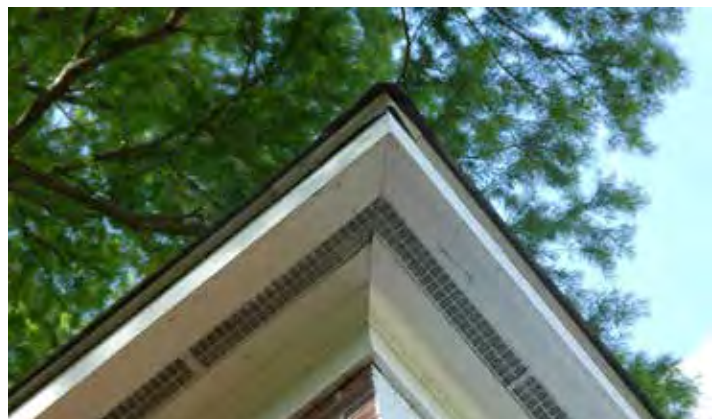
Soffit vent at one-story 1960s addition
