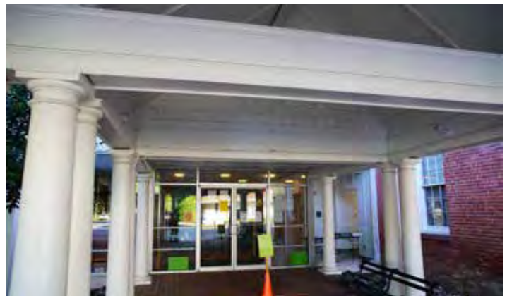
Single-pane aluminum storefront entry is partially sheltered by breezeway
