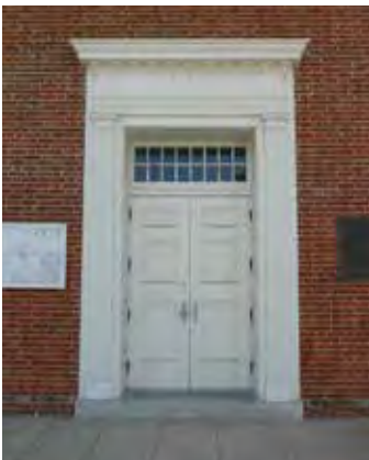
Painted wood door surround in good condition
