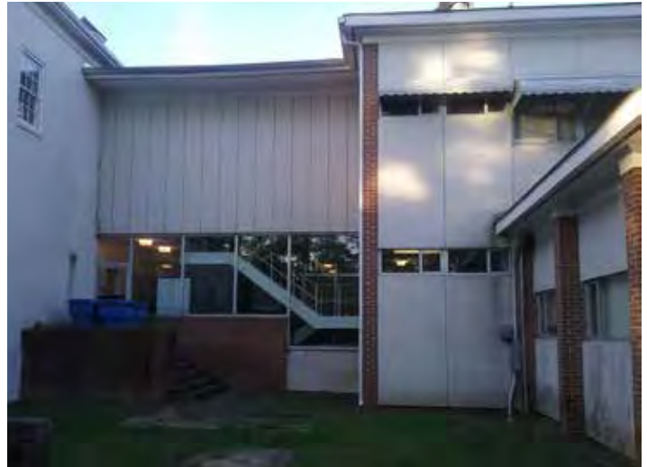
Precast panels at 1960s addition
