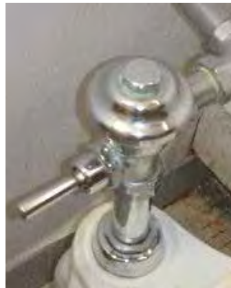
P.3 – Water damage, Witness Room restroom
