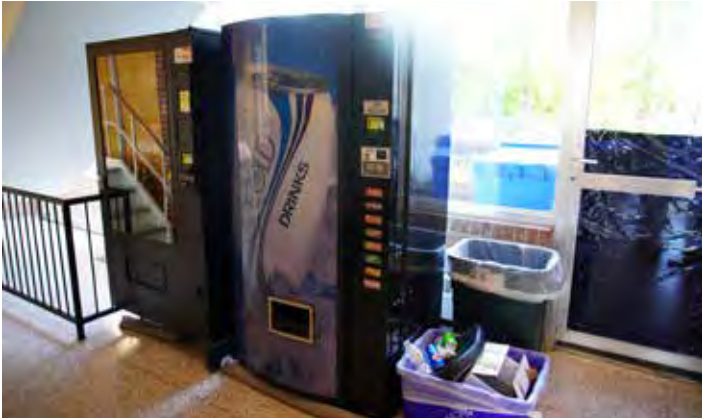
Equipment and refuse storage in stairwell; code-compliant cane detection rail is present below stair (left)
