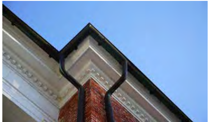
Gutters, downspouts, and painted wood cornice in good condition
