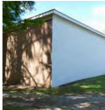
Painted and unpainted brick at SW corner of one-story 1960s addition
